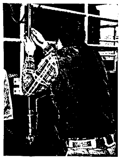
Technician using Pitometer rod in Waltham Pump Station.
