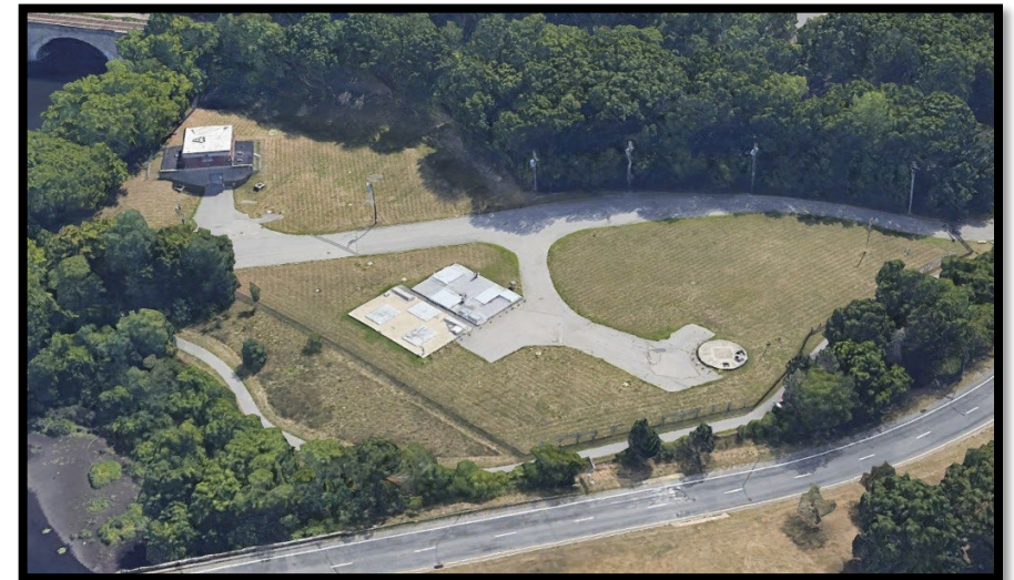
Shaft Site After Construction
