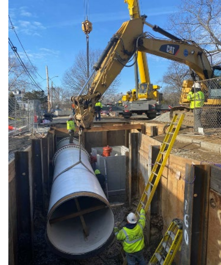
WASM 3 – pipe replacement
